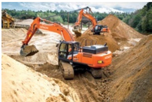
Zaxis medium excavators
