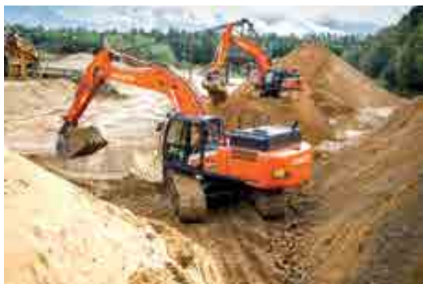
Zaxis medium excavators
