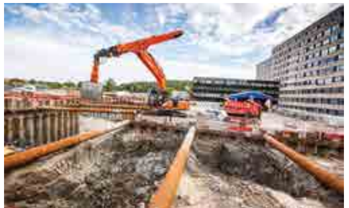
Special application excavators
