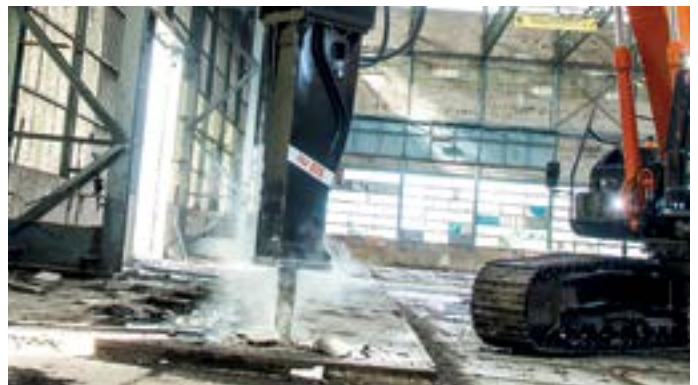
Breakers are lightweight with high impact energy.
